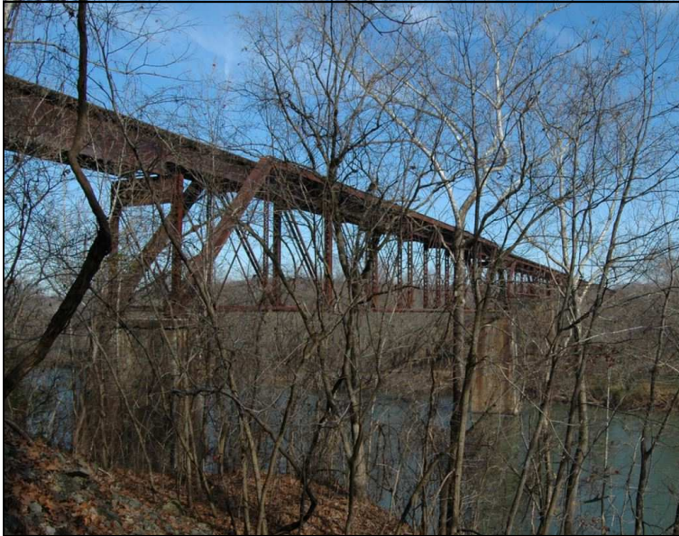
The Rock Island trestle spanning the Gasconade River valley, at nearly a mile long and one hundred feet high, presents a daunting challenge to park builders and eventually to those who wish to walk or ride over it.
